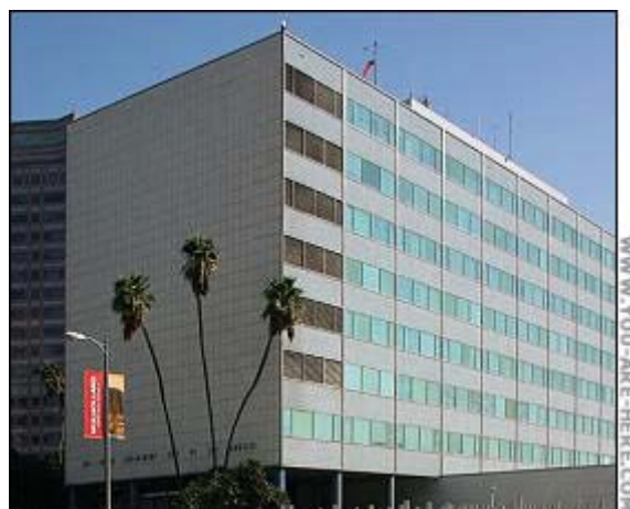
Building: Los Angeles Police Department
